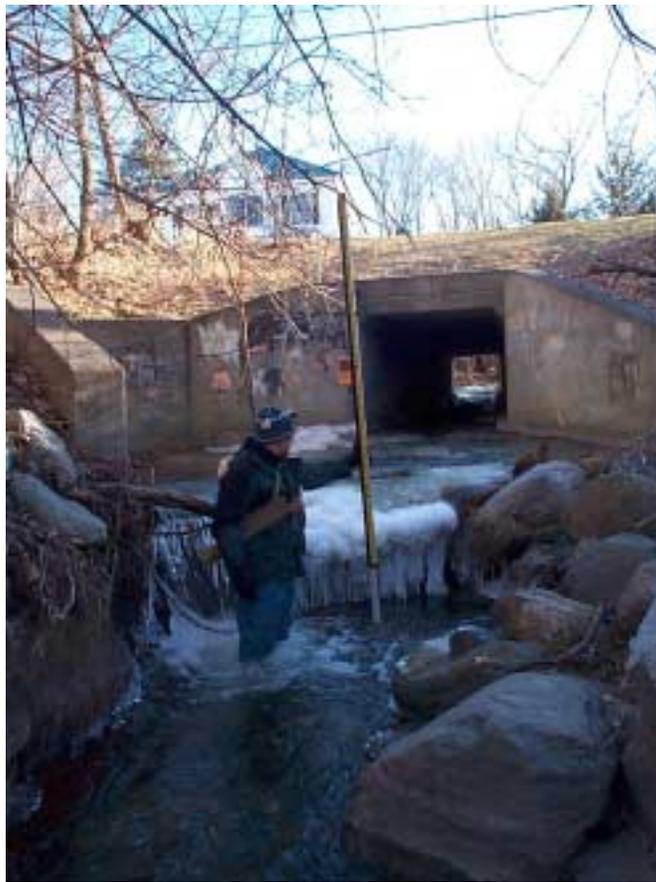
Upstream view of the Lincoln St. culvert. At the time it was constructed the streambed was level with the invert of the culvert. Note that within the past few years the bed has degraded approximately 3 feet.
